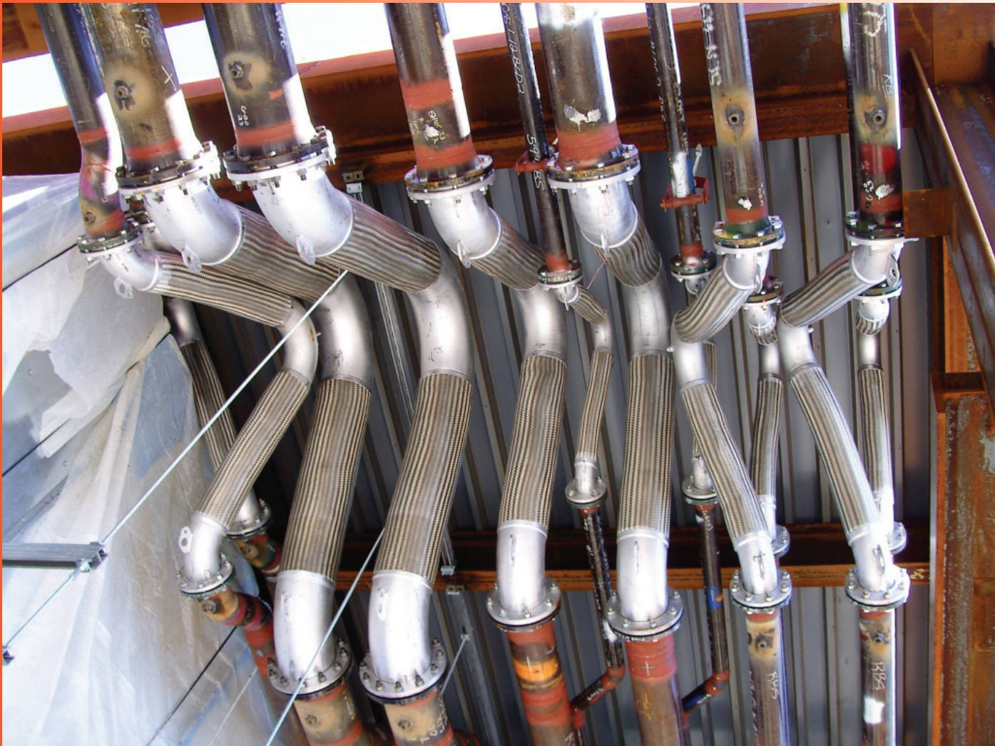
VERTICAL VFL INSTALLATION (Apex Near Ceiling)
