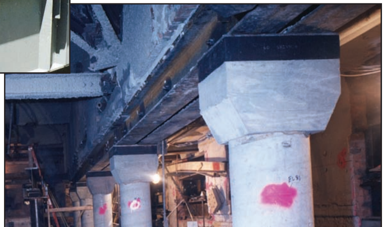
Subway Isolation Pads Under Carnegie Hall
