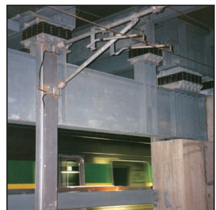
Train Passing Immediately Adjacent to Building Columns- Note Spring Isolation on Top of Column
