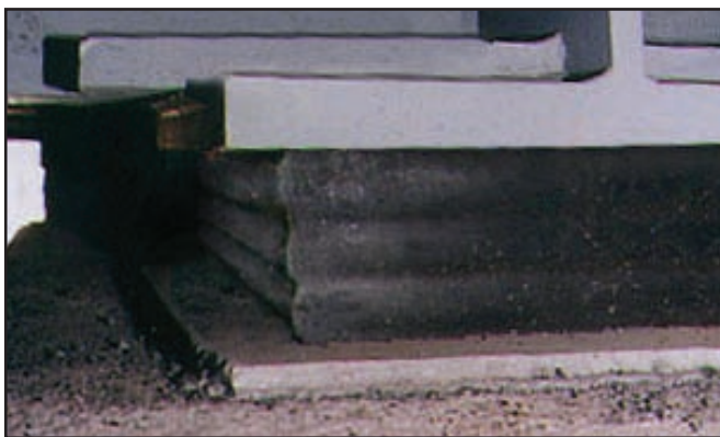
Loaded Bearing Showing Bulges Between Plates
