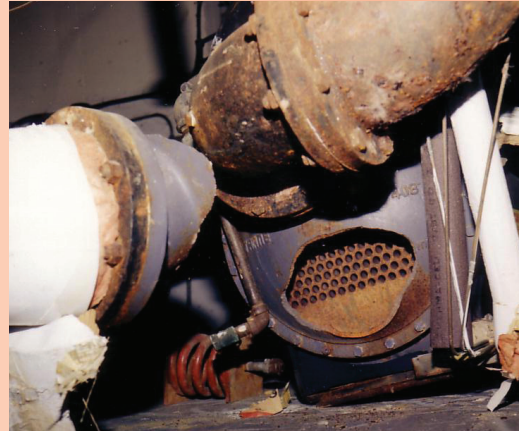
Lack of Flex Connector Caused Cast Iron Failure
